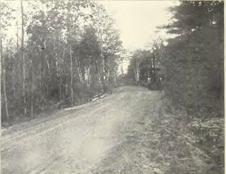
A Piece of Road through the Forests completed
